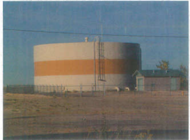
Water Storage Tank in Belen
