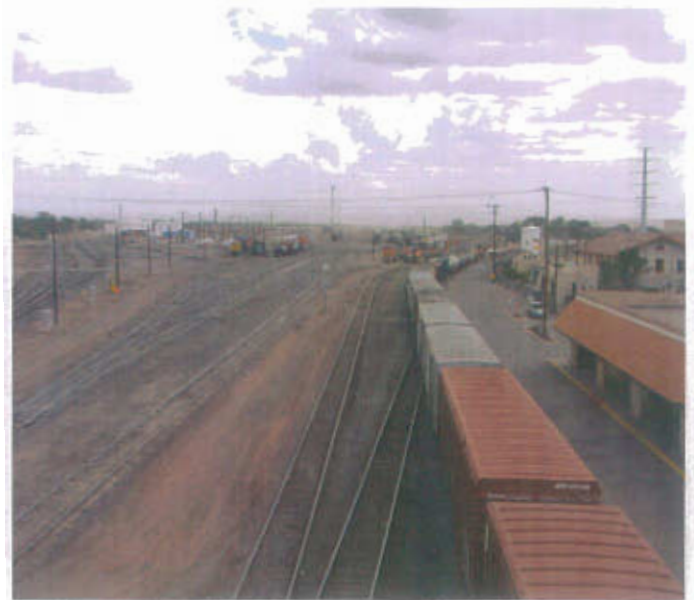
Belen Rail yard
