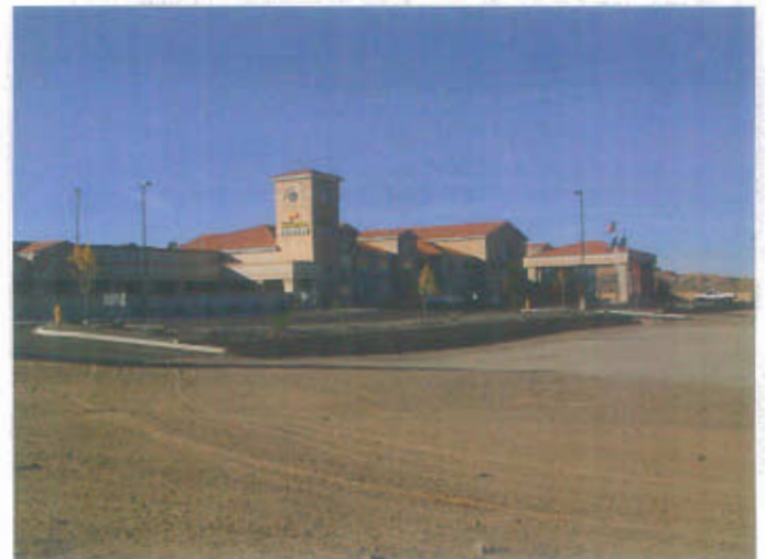
Holiday Inn at West Belen Interchange
